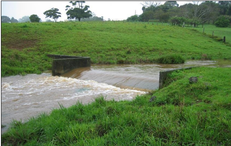
Image 2 – Typical stable rock control
